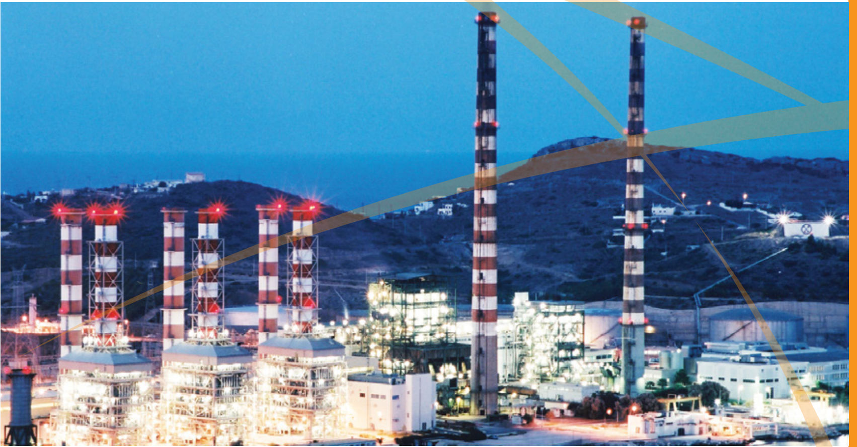
Public Power Corporation Power Plant (Lavrio of Attica)
