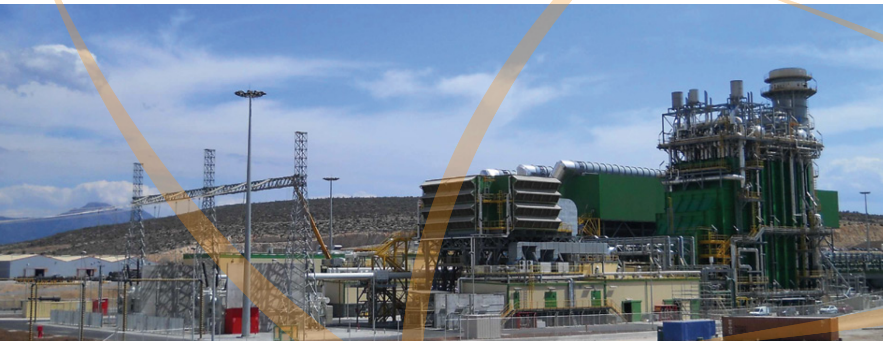
ELPEDISON Power Plant
