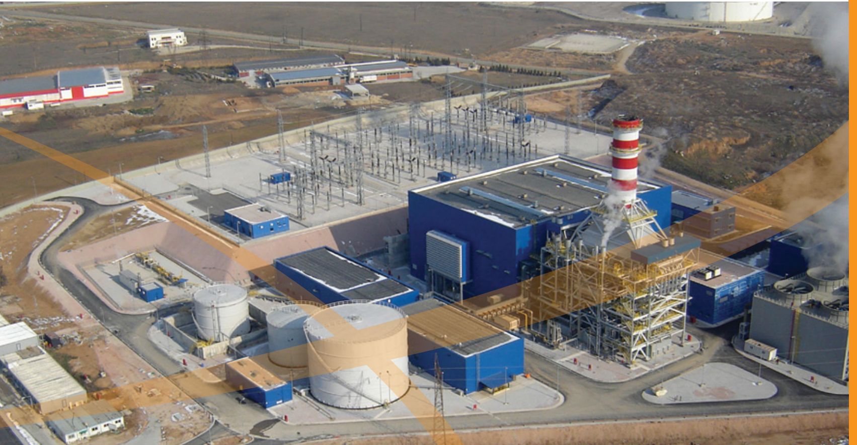
ELPEDISON Power Plant (Station in Thisvi of Viotia)
